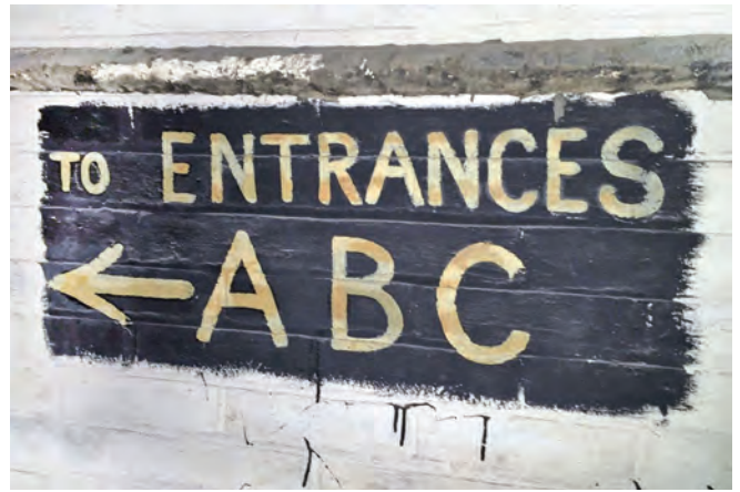
WWII signage survives in the tunnels. Photo Ian Walker
